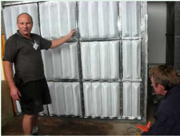
Rodney proudly discusses the completed installation while they admire the work.
